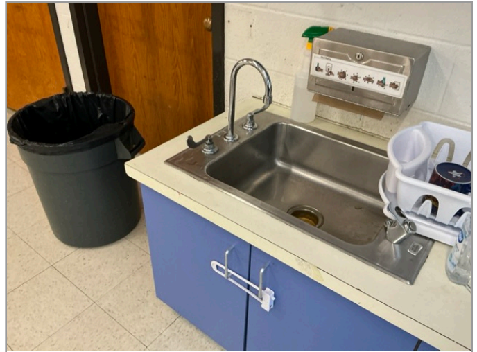
SINK CLEARANCE (SIDE APPROACH)
