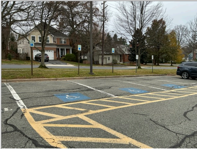
OVERVIEW OF ACCESSIBLE PARKING AREA
