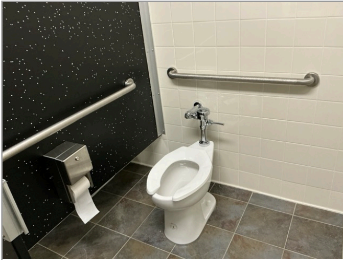
TOILET STALL OVERVIEW
