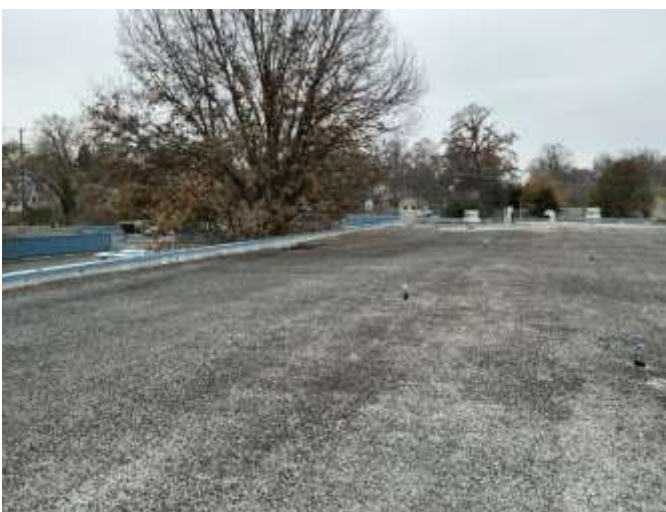
5 - PRIMARY ROOF OVERVIEW
