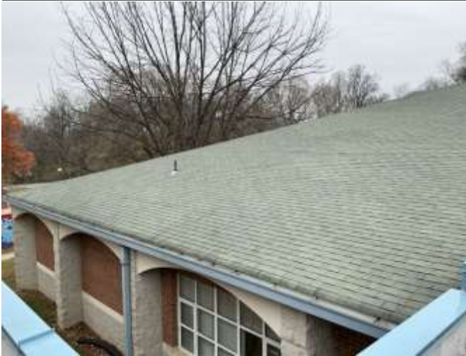
7 - SECONDARY ROOF OVERVIEW
